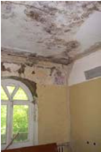
Sampling room ceiling
